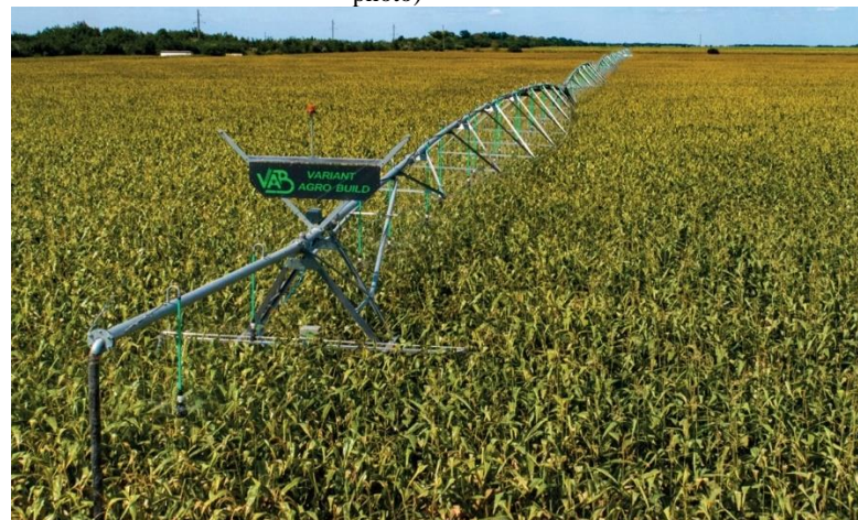
Fig. 8. Pivot irrigation system at Agro Mares SRL (original photo)
