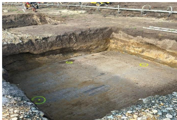
Fig. 9 Pouring the leveling concrete after leveling
