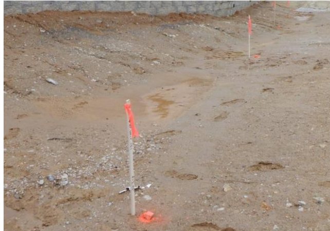
Fig. 8 Road border stakeout using 3d line stakeout method
