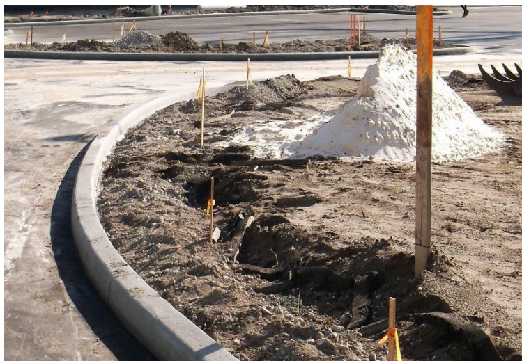
Fig. 7 Pedestrian Road stakeout using Arc stakeout method
