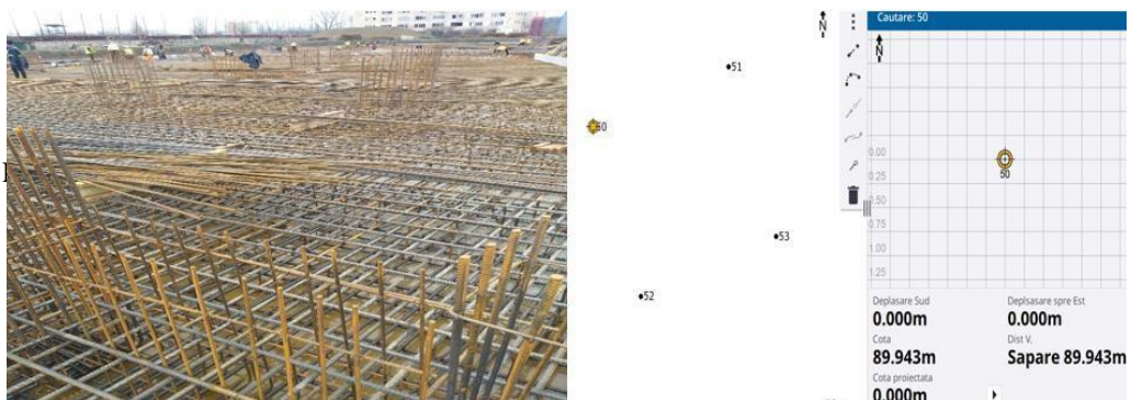
Fig. 5 Point stakeout method to determine pillar corners
