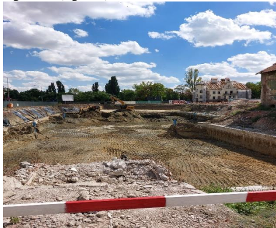
Fig.5 Realization of the excavation, of the volume
