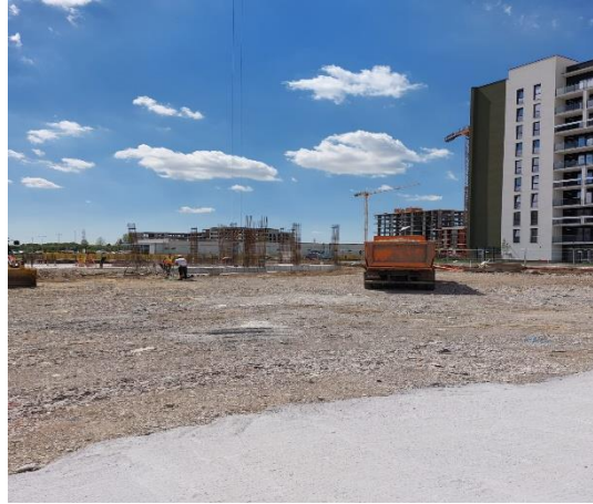
Fig.6 Elevation 0.00 and the structural elements of the future residential building
