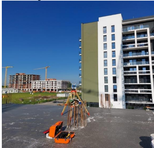
Fig.7 Plotting construction elements with the Stonex R35 total station
