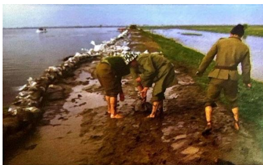
Figure 1. Dyke protection work (source: Romanian Waters)
