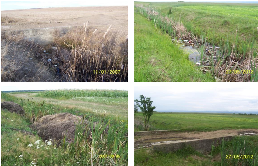
Figure 6: Clogged culvert showing vegetal and household residue within the canals
