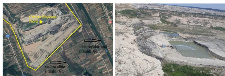
Figure 4 Old Jiu river bed crossing the North Pesteana mining perimeter (left);The location of the sumps on the base of the North Pesteana pit (right)
