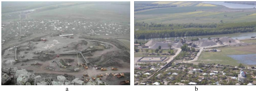
Fig. 2. Crushing plant and loading Dock
