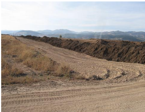
Figure 1 - Land prepared for excavation
