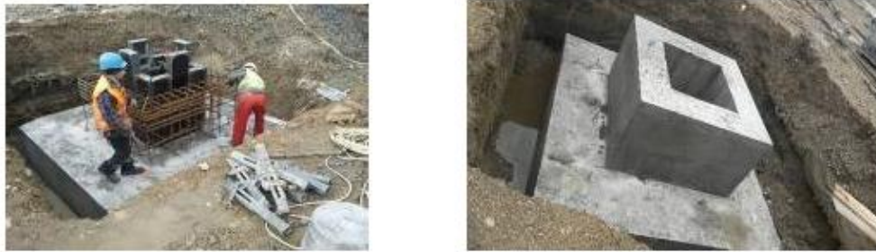
Figure 7-8 The foundation base and the foundation collar.
