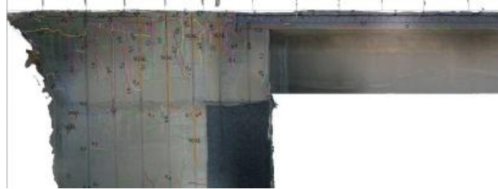
Figure 7. Digitized cracks and pathology on the orthomosaic of the bridge
