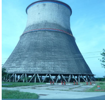
Figure 1: The cooling tower from the area of CET Timișoara South
