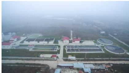
Fig. 3. Călărași wastewater treatment plant
