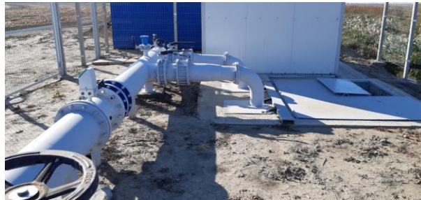
Photo 6 Realization of the annex constructions for concrete tank type stations
