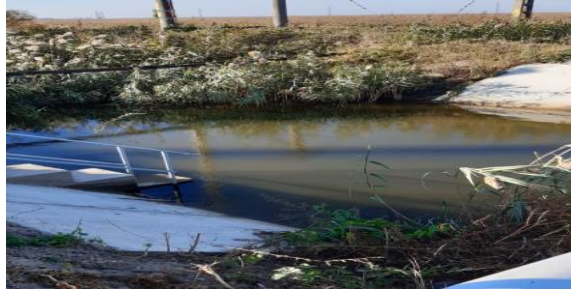
Photo 7 Protecting the canal in the suction area
