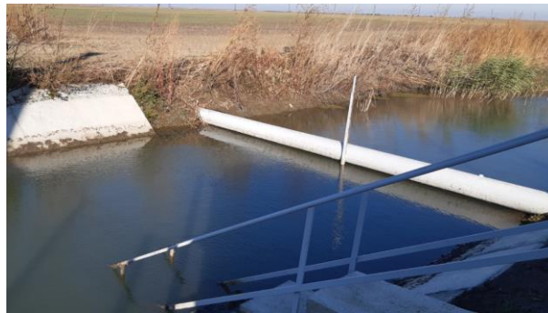
Photo 8 Crossing the pipe to the antenna
